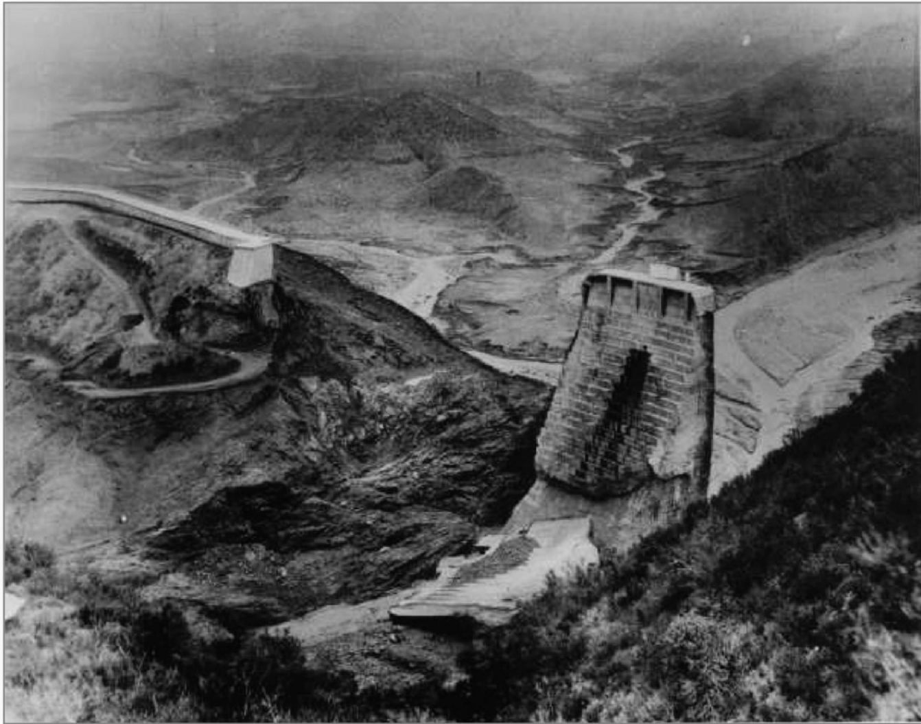
St. Francis Dam, 29 March 1928
