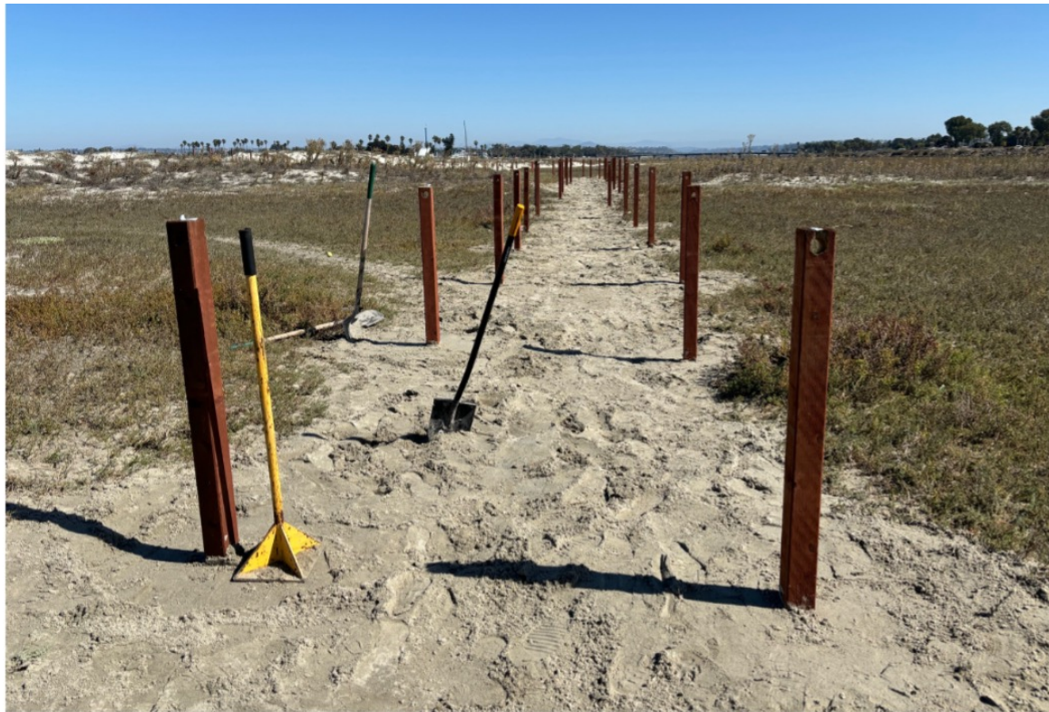
Photo 2.2. Fencing installation in Q4 2024
