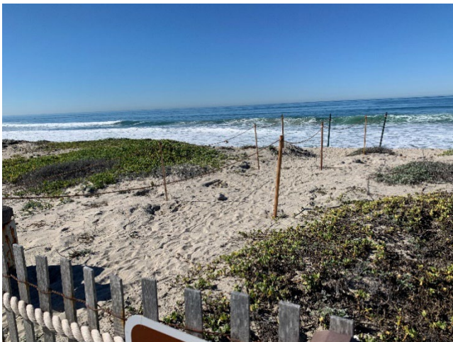
Photo 5. Fence installation for beach access
