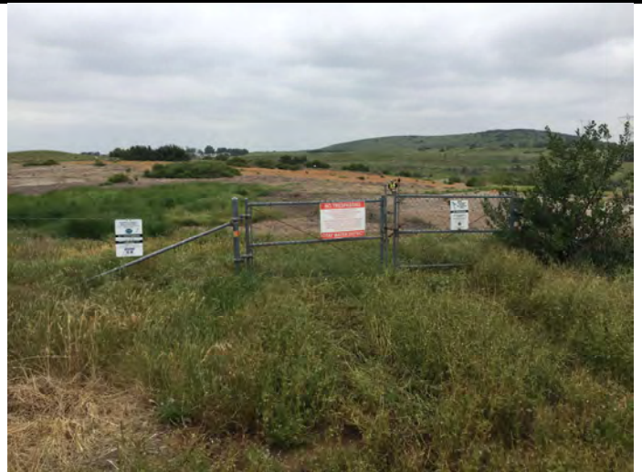
Photo 14 – Illegal Entry Point East 3b. After installation of site deterrents: new signage on perimeter fence and cell-enabled camera in background at Burrowing Owl burrow (see Photo 15)). Date: 4/12/2024 and directed west.
