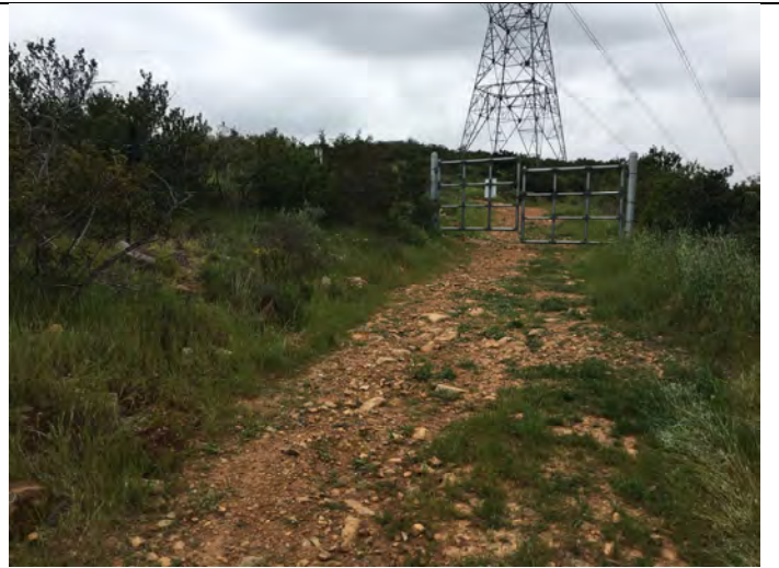
Photo 2 – After installation of all site deterrents: new gate, cell-enabled project monitoring camera (along the edge of the trail), new signage, and cactus cuttings. Date: 4/12/2024.
