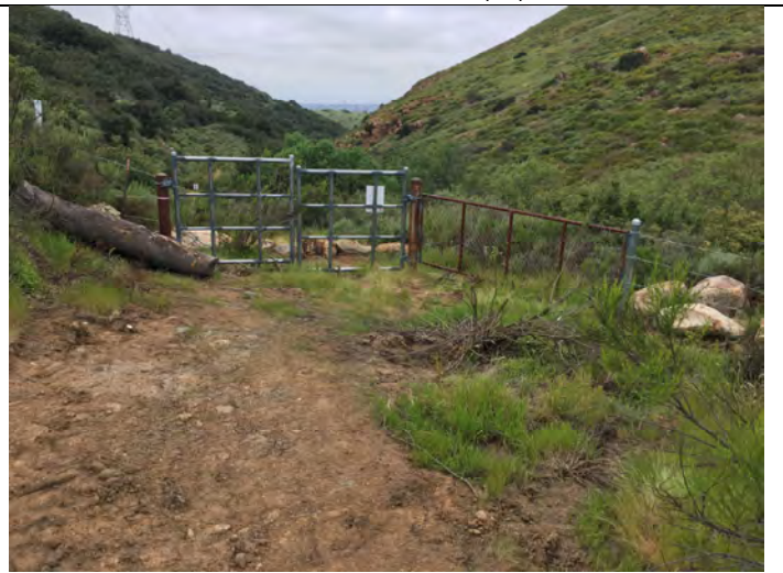
Photo 6 – After installation of all site deterrents: new gate, cell-enabled project monitoring camera (along the edge of the trail), new signage, and cactus cuttings. Other perimeter repairs were completed as part of the regular HMA responsibilities (not funded by the Grant). Date: 4/12/2024.
