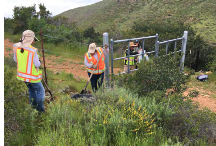
Photo 3 – Illegal Entry Point West 1b. Installation of deterrents. Date: 4/12/2024 and directed north.
