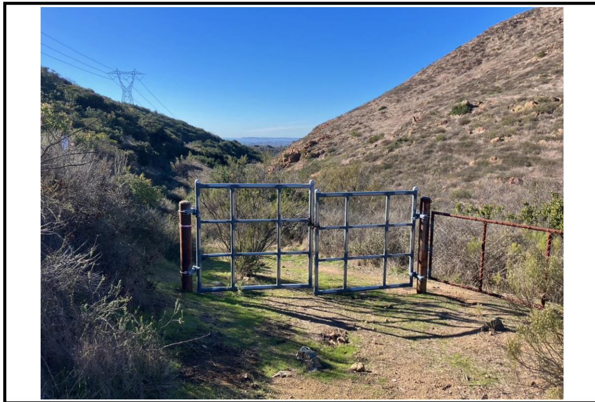
Photo Point 2. Illegal Entry Point West 1a. Installation of new gate. Photo date: 1/9/2024. During installation of the new gate, the original gate was shifted to the north (right of the new gate) in hopes that it would deter trespassers from cutting the barbed wire fence adjacent to the new gate. Unfortunately, trespassers cut the barbed wire fence to the left of the new gate and are continuing to cut the fence to the right of the gate (out of view).
