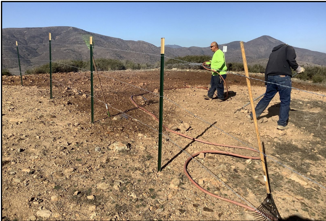
PHOTOGRAPH 13 Seed was Raked into the Soil and Watered to Help the Seed Stick to the Soil, December 7, 2023
