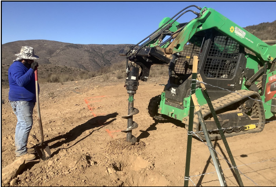
PHOTOGRAPH 31 Digging Holes for the Bollards Using the Skid Steer Mounted Auger, November 9, 2023
