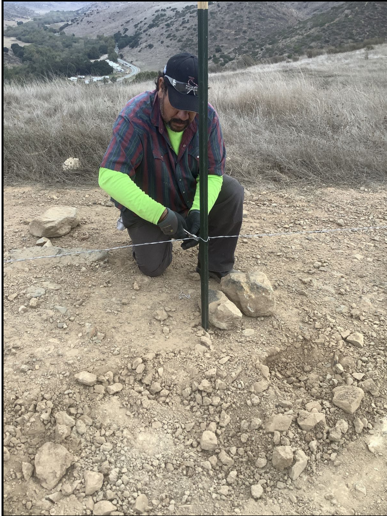
PHOTOGRAPH 35 The Crew Securing the Fence Wire with a Tie, November 7, 2023
