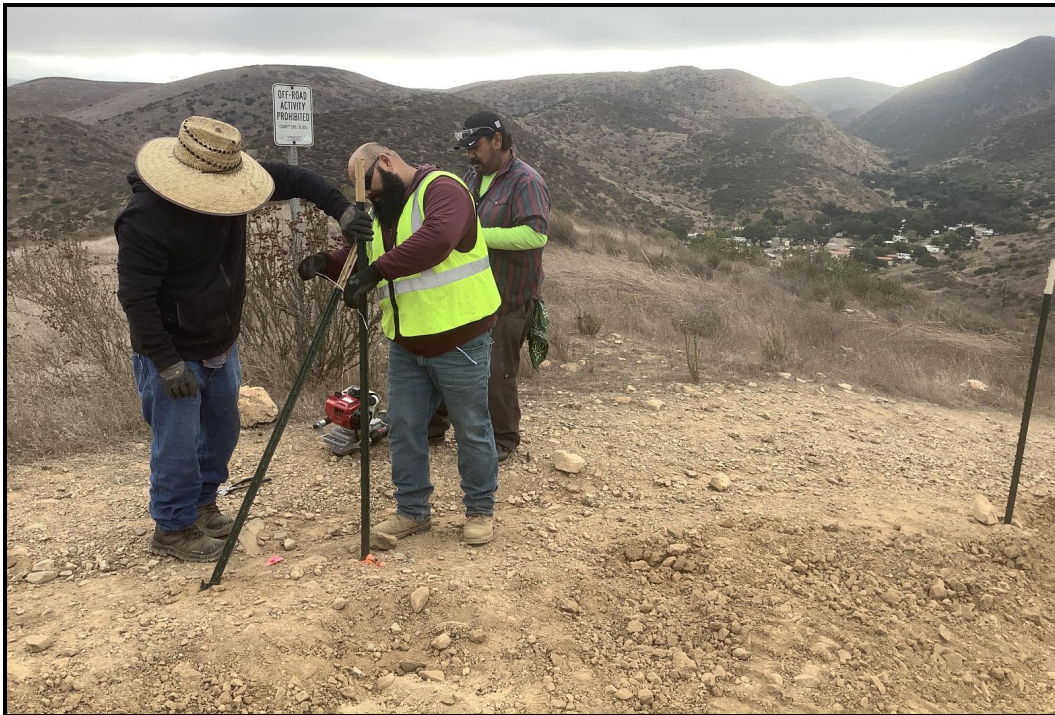
PHOTOGRAPH 34 The Crew Securing Angled Braces Before Stringing Wire Fencing, November 7, 2023
