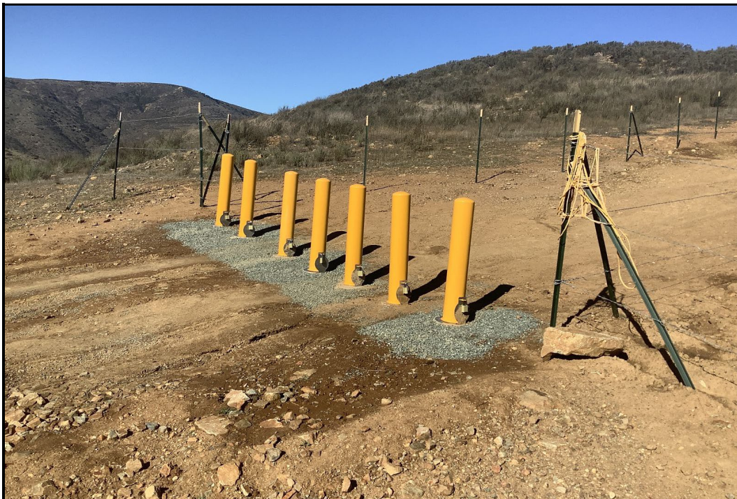
PHOTOGRAPH 32 The Removable Bollards Were Installed in Their Bases and Locked, January 12, 2024
