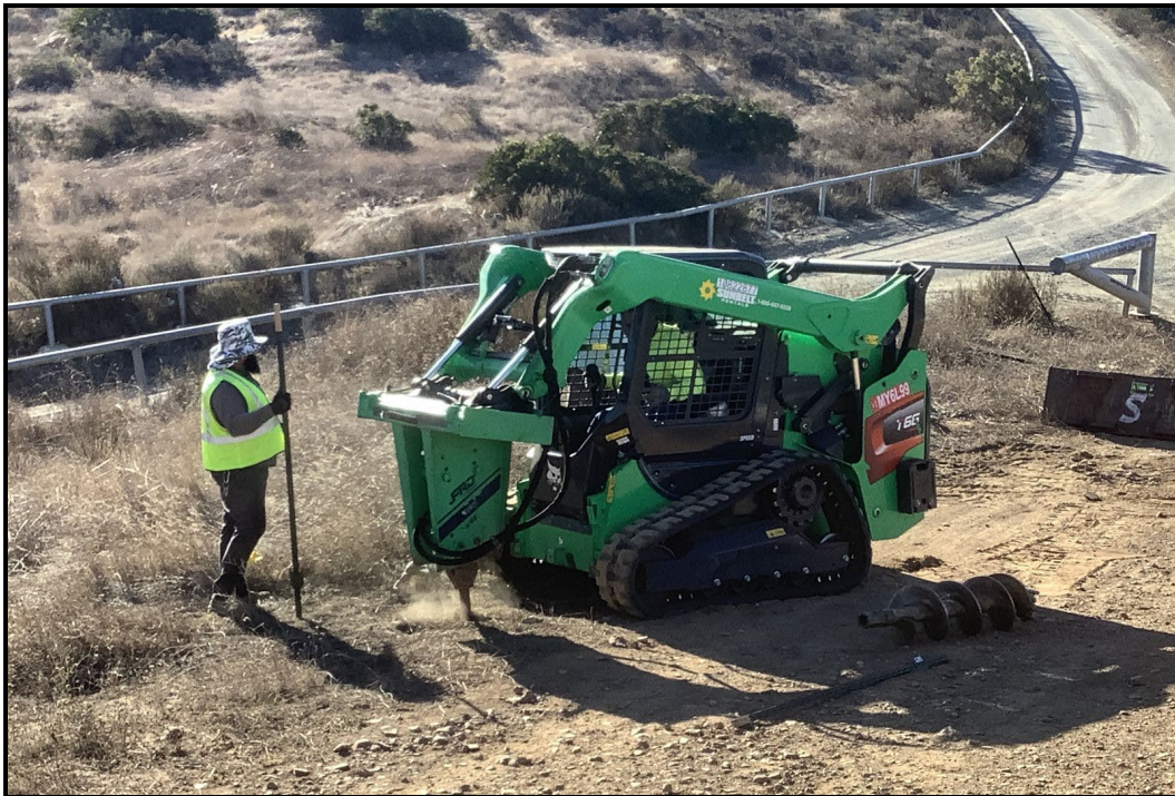
PHOTOGRAPH 37 A Jackhammer Attachment on the Skid Steer Was Used to Drill Holes for the T-posts, November 6, 2023
