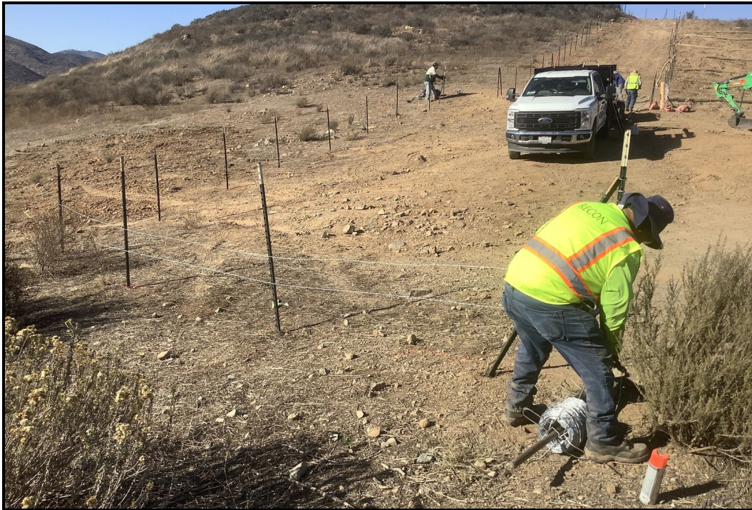
PHOTOGRAPH 36 The Crew Pulling the Fence Wire Tight, November 9, 2023
