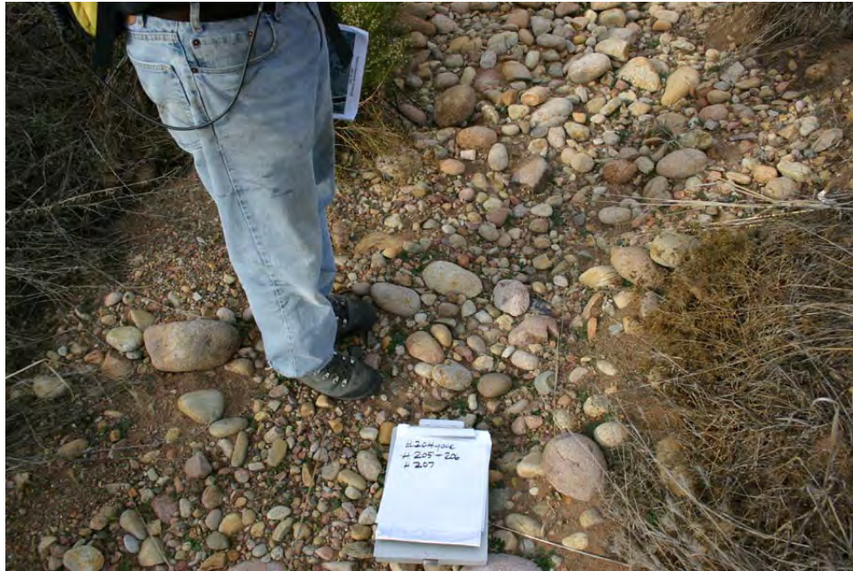
Plant (207) – Missing, scour.
