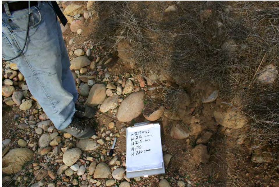
Plant (210) – Missing, scour.
