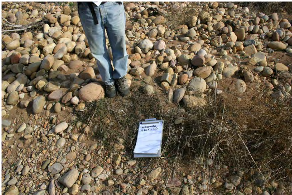
Plants (223 & 224) – Missing, scour.
