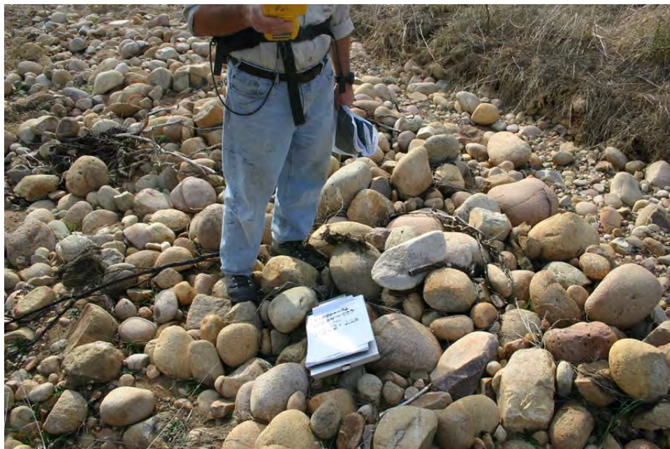
Plants (222 & 225) – Missing, scour.
