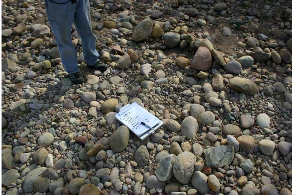
Plant (264 & 263) – Missing, scour.
