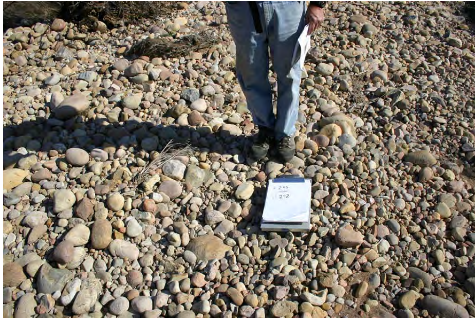
Plant (292) – Missing, scour.
