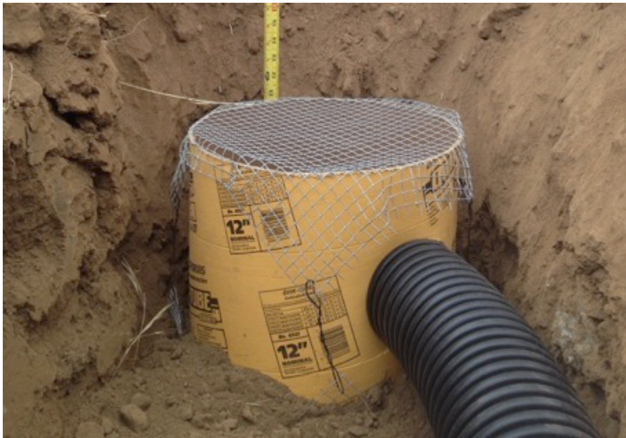
b) Below-ground chamber of acclimation burrow made of concrete form tubing.
