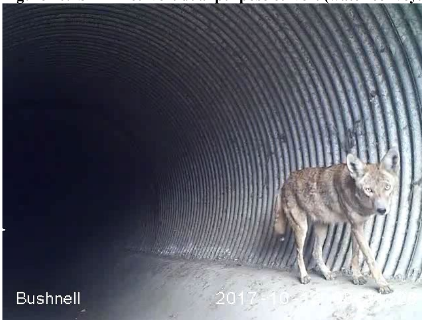
Figure 20. SR 241 culvert dual purpose culvert (water conveyance and wildlife undercrossing)
