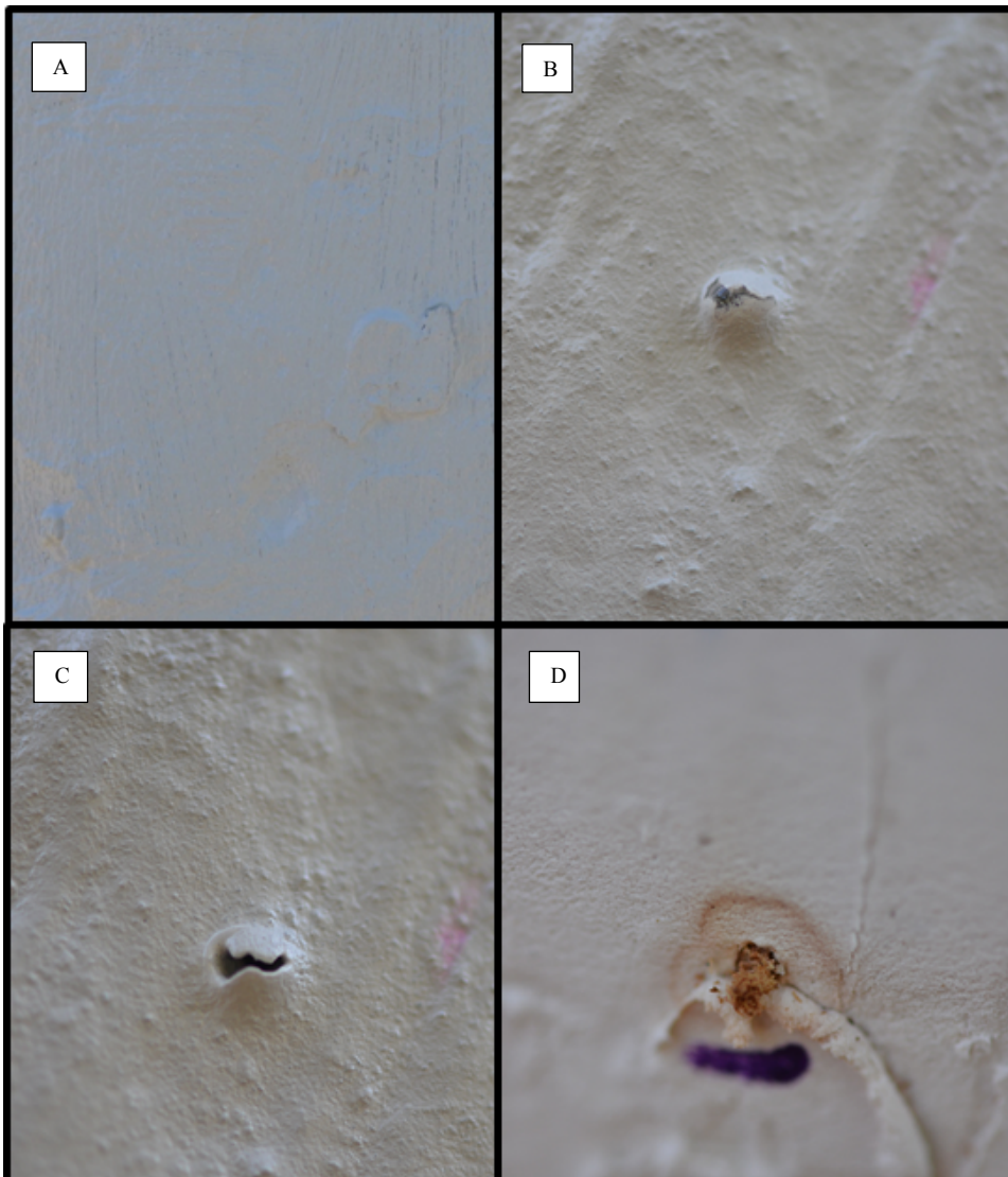
Figure 14. Progression of beetle reemergence in after paint application. After paint application has begun to dry (A), the female beetle will begin re-establish the entry point with her abdomen (B), break through the paint obstruction (C), and continue to maintain the gallery (D).
