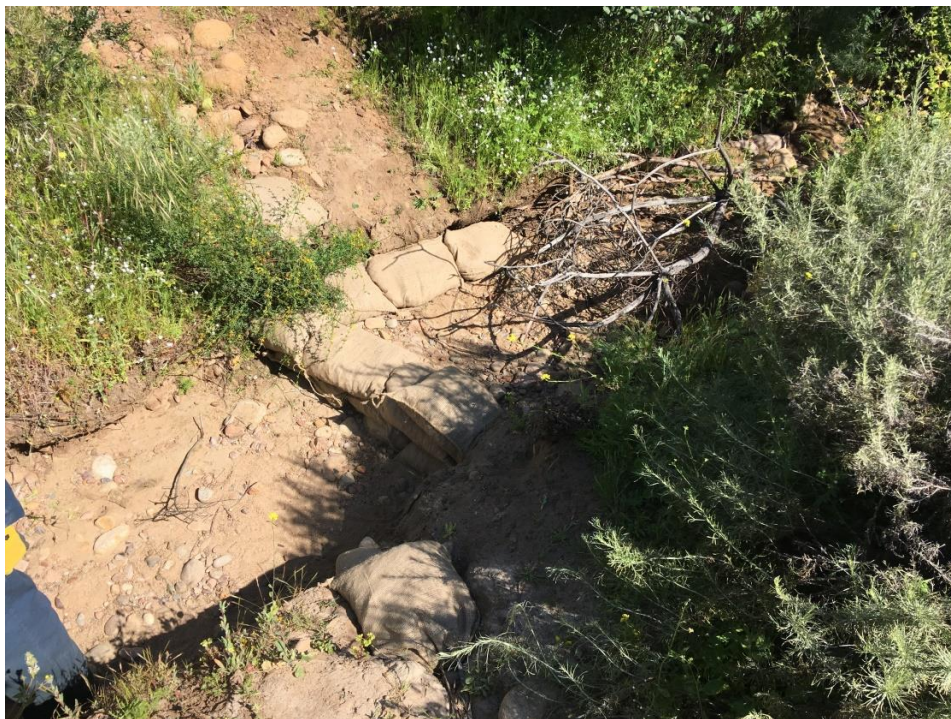
Terrestrial Site 2- view of erosion control measures & vertical mulch – July 2019
