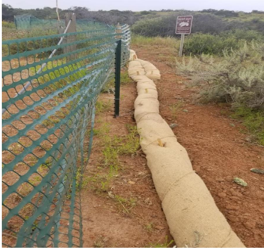
Representative view of installed fiber rolls July 2019
