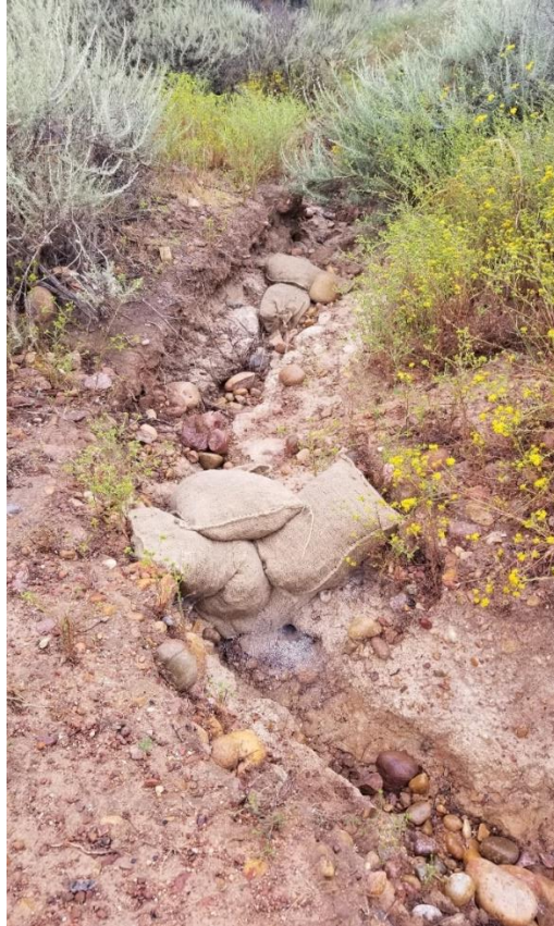
Terrestrial Site 2- view of erosion control measures & vertical mulch July 2019
