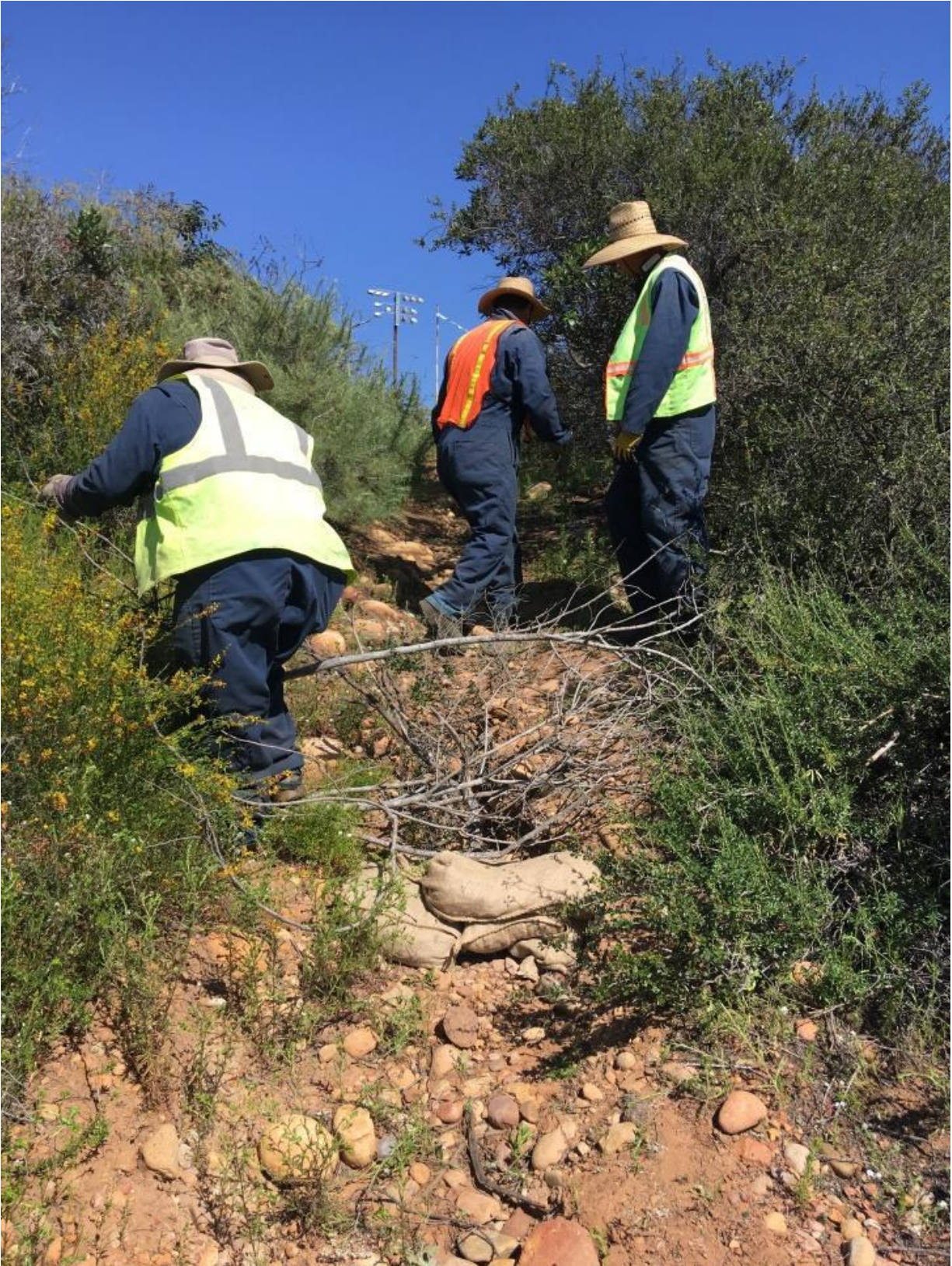
Representative view of gravel bag check dam & vertical mulch. July 2019
