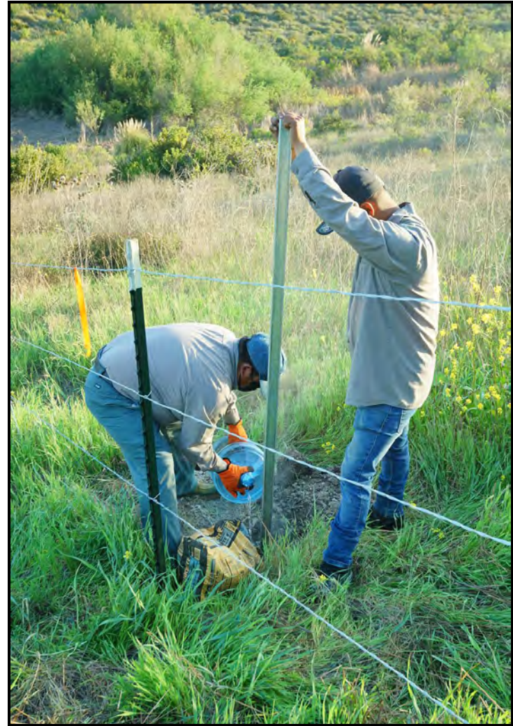
PHOTOGRAPH 7 RECON Crew Cementing in New Signpost in Rice Canyon–April 2021
