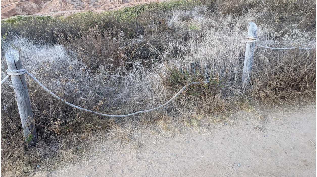
Broken and worn post and rope before replacement (Photo Credit: P. Geisler)
