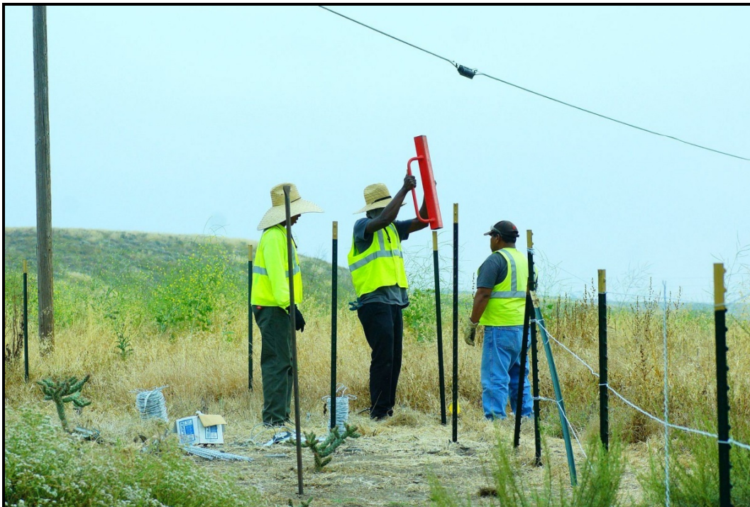
PHOTOGRAPH 10 RECON Crew Installing Fence April 2017
