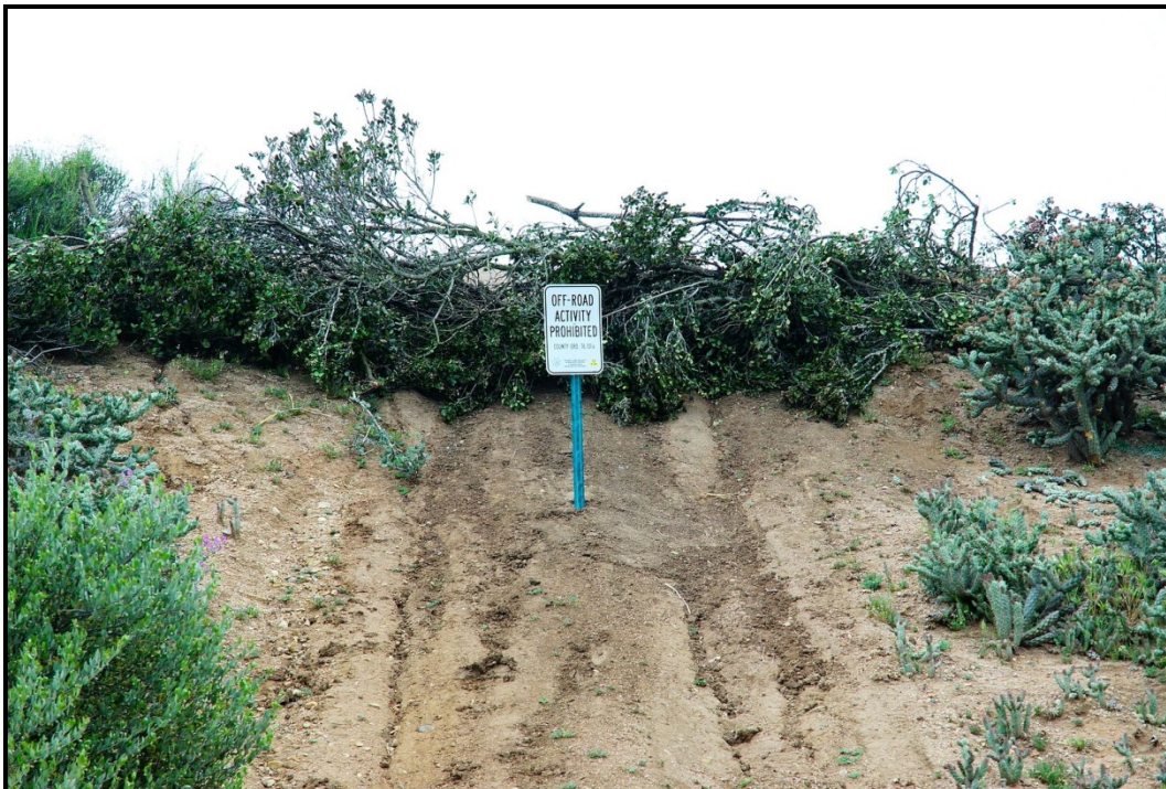
PHOTOGRAPH 4 Lemonadeberry Branches were Placed on the Slopes to Block Motorcycle Trails
