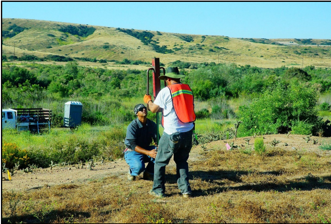
PHOTOGRAPH 9 RECON Crew Installing Fence April 2017
