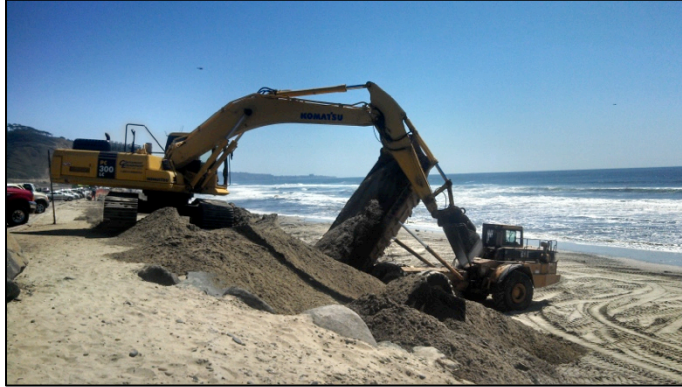
Figure 18. Dumping excavated sand along the eroded bluff used for the heavy equipment staging area. Photo by Mike Hastings.
