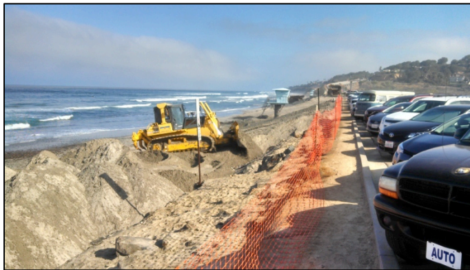
Figure 23. Re-contouring sand piles placed along the eroded bluff adjacent to N. Torrey Pines Road. Photo by Mike Hastings.
