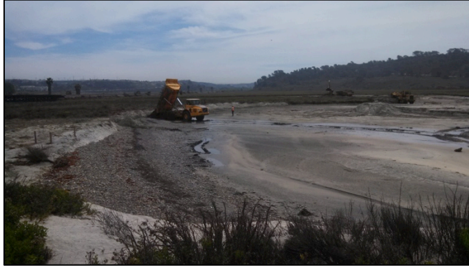
Figure 21. Placing excavated spoils along the eroded embankment to restore the remnant dune area eroded over the previous years. Photo by Mike Hastings.
