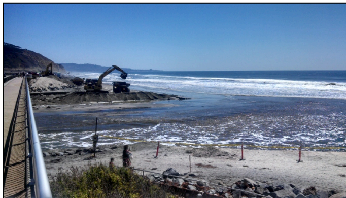
Figure 17 Excavating the channel between Transect A1 and Transect A2. Photo by Mike Hastings.
