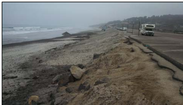
Figure 60. Soft-armoring of N. Torrey Pines Road and improved public access/safety using sand removed from the inlet at Los Peñasquitos Lagoon. Photo by Mike Hastings.
