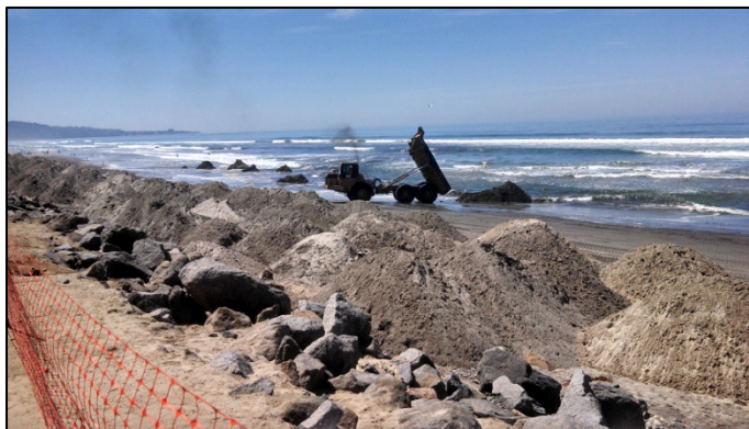
Figure 20. Placing excavated spoils along the waterline on Torrey Pines State Beach. In the foreground are sediment piles placed in front of the eroded bluff along N. Torrey Pines Road. Photo by Mike Hastings.
