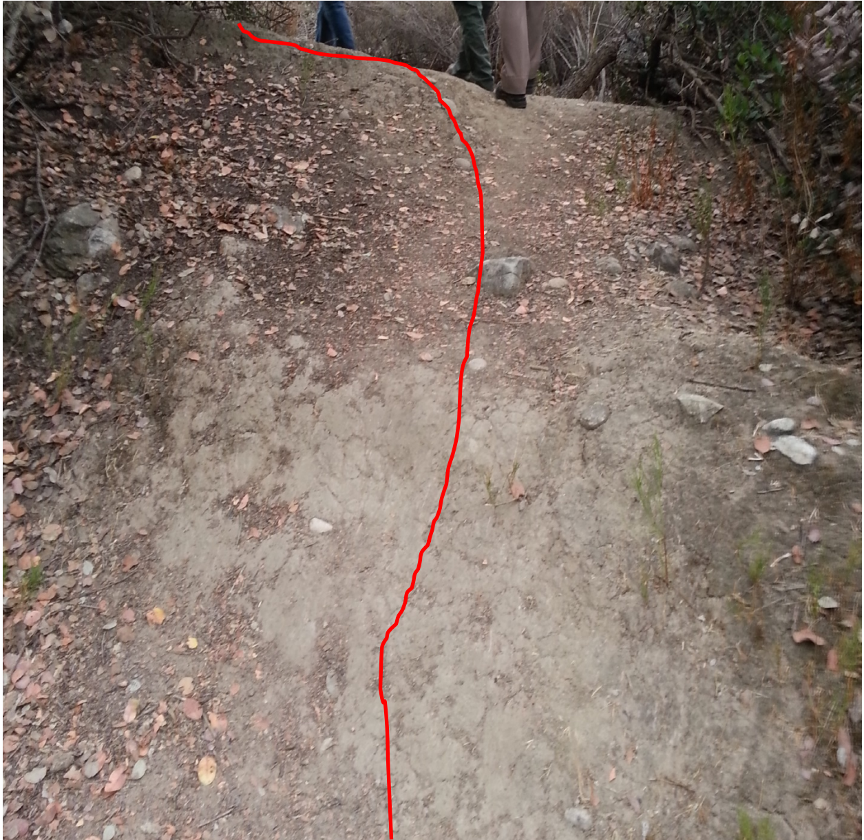
Photograph 5: Emerald Hills Canyon, facing southwest toward bend in the trail up to Bethune Court trail head. Photo shows very steep, eroded trail to be refurbished.
