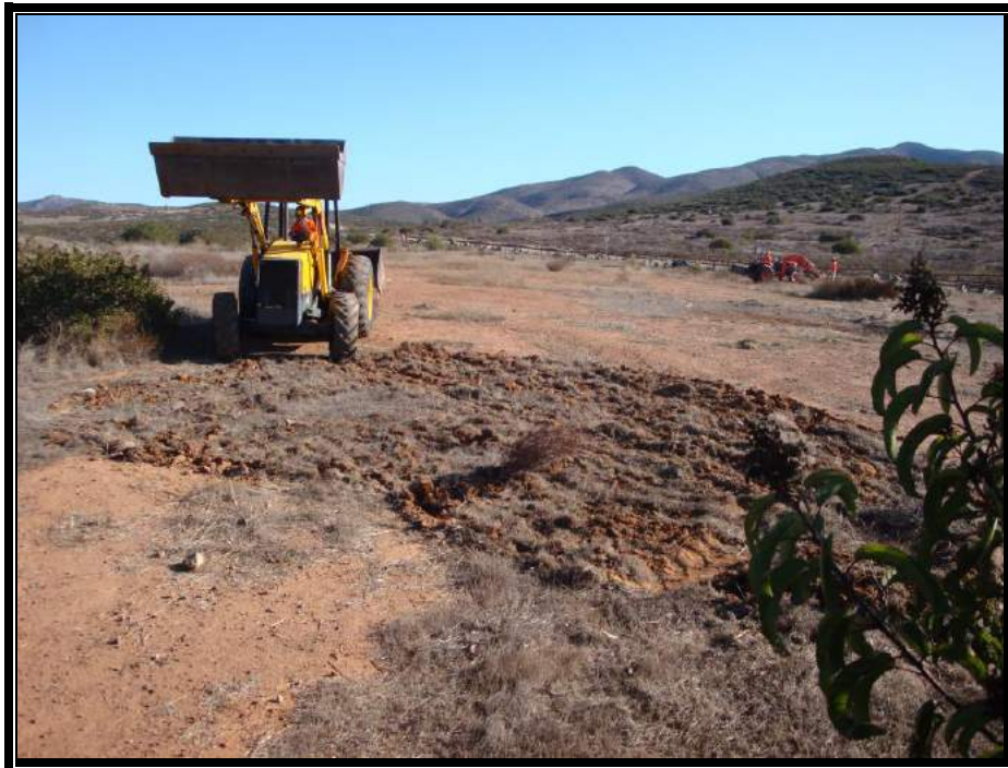
Contractors grading constructed vernal pools.
