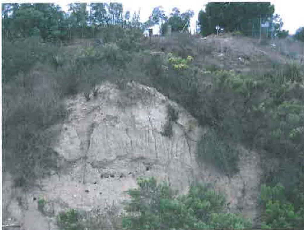
20. Scour through the embankment of a historical detention basin near the landfill. - Looking West
