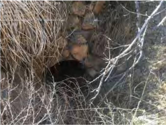
westbound: Small culvert east of this location. This is culvert entrance on north side. The culvert exit on the south side of 76 is not accessible.
