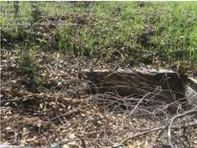
northbound Blocked, small diameter culvert entrance
