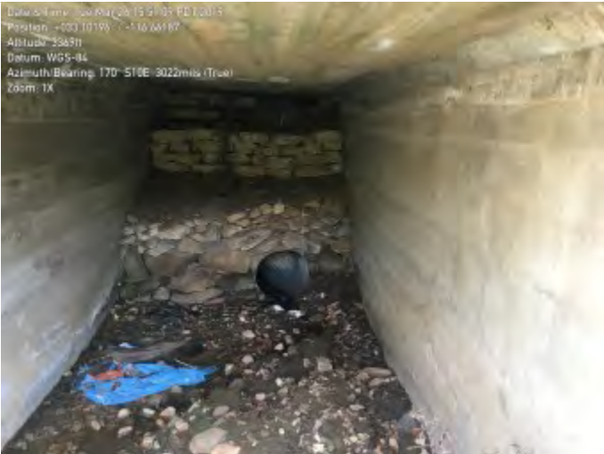
westbound Entrance to culvert which transitions to small diameter pipe culvert
