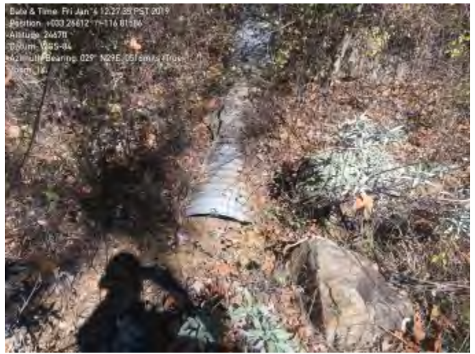
eastbound blocked culvert exit
