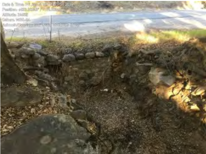
eastbound blocked culvert
