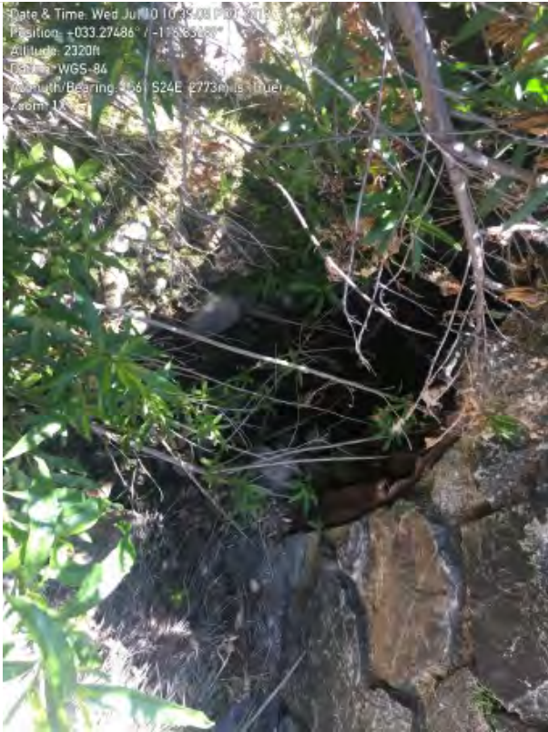
westbound partially blocked culvert entrance
