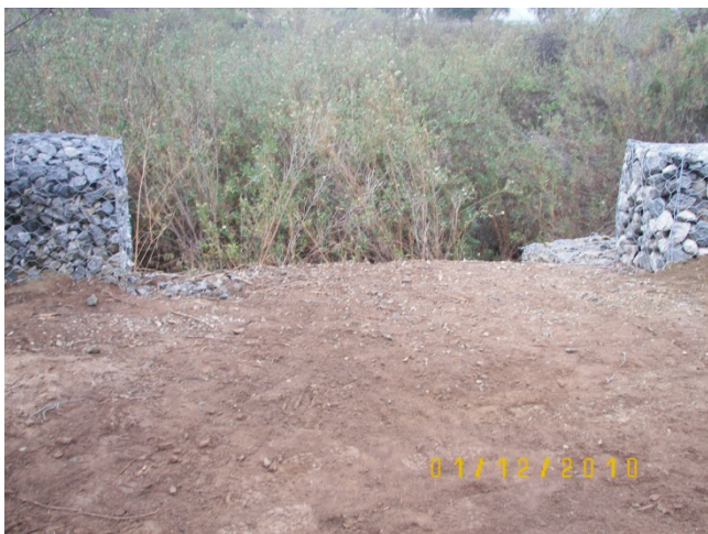
Photograph 5: Repaired gabion baskets in CE 3 showing where water will flow.
