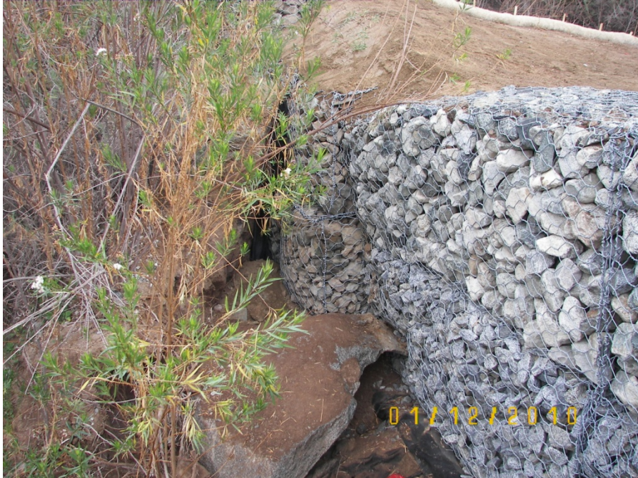
Photograph 5: Gabion baskets and area where water lands during flow events.
