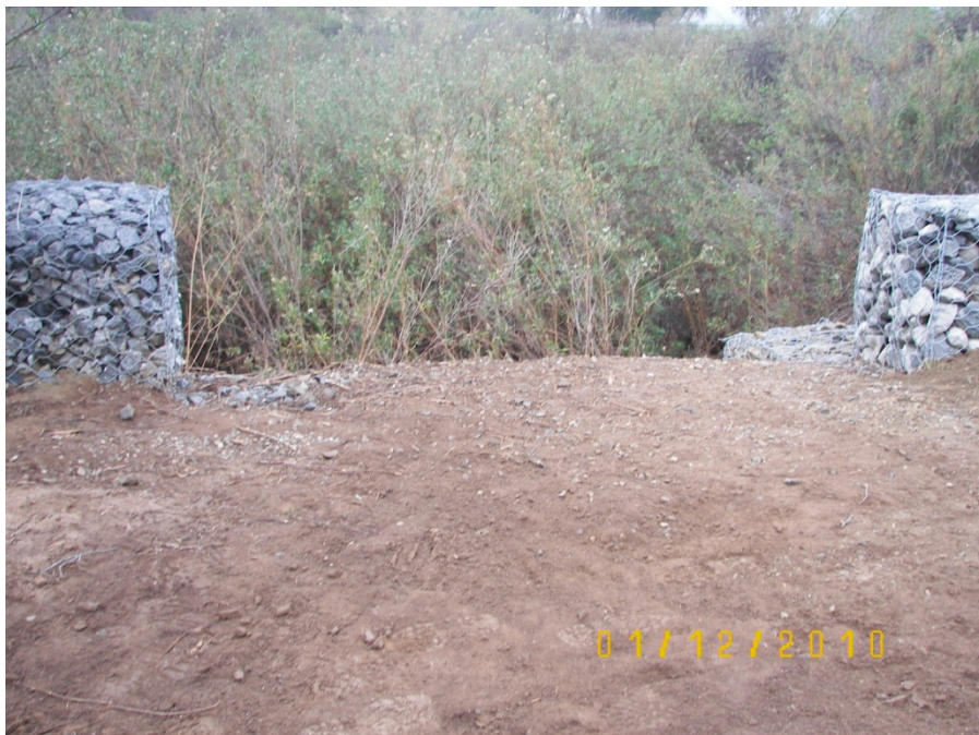
Photograph 3: Gabion baskets and water outlet.
