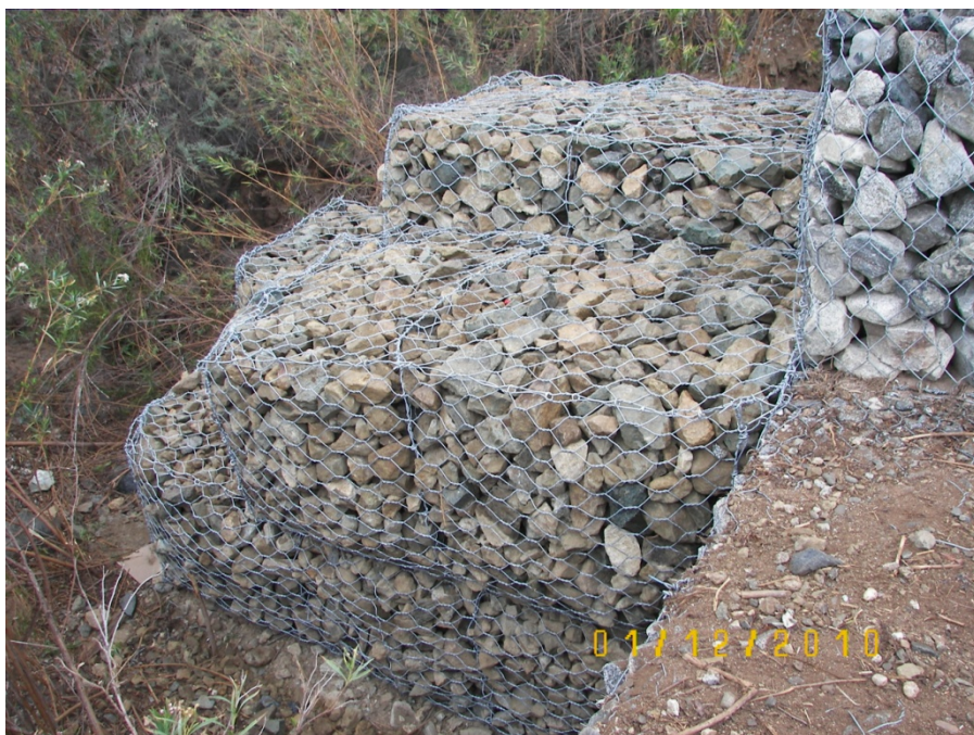
Photograph 4: Gabion baskets, up close.
