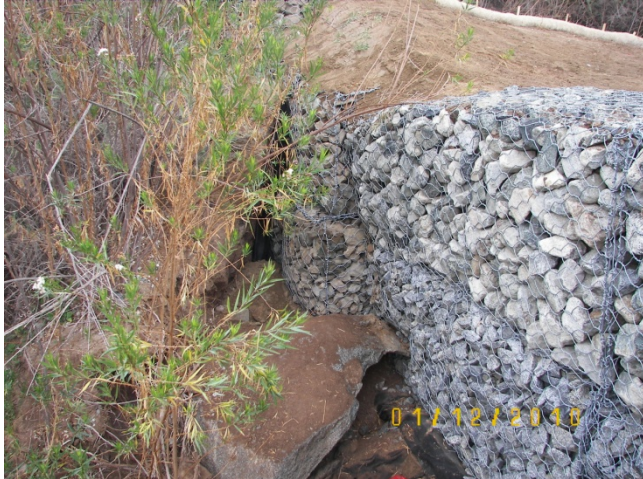
Photograph 3: Repaired gabion basket in CE 3.
