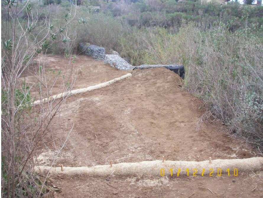
Photograph 1: Erosion control devices and gabion baskets, looking south.
