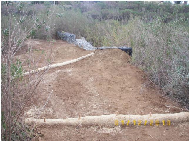
Photograph 4: Repaired gabion baskets with erosion control in CE 3.
