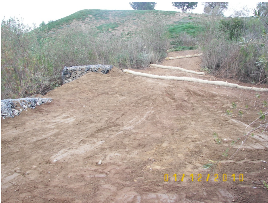
Photograph 2: Erosion control devices and gabion baskets, looking north.
