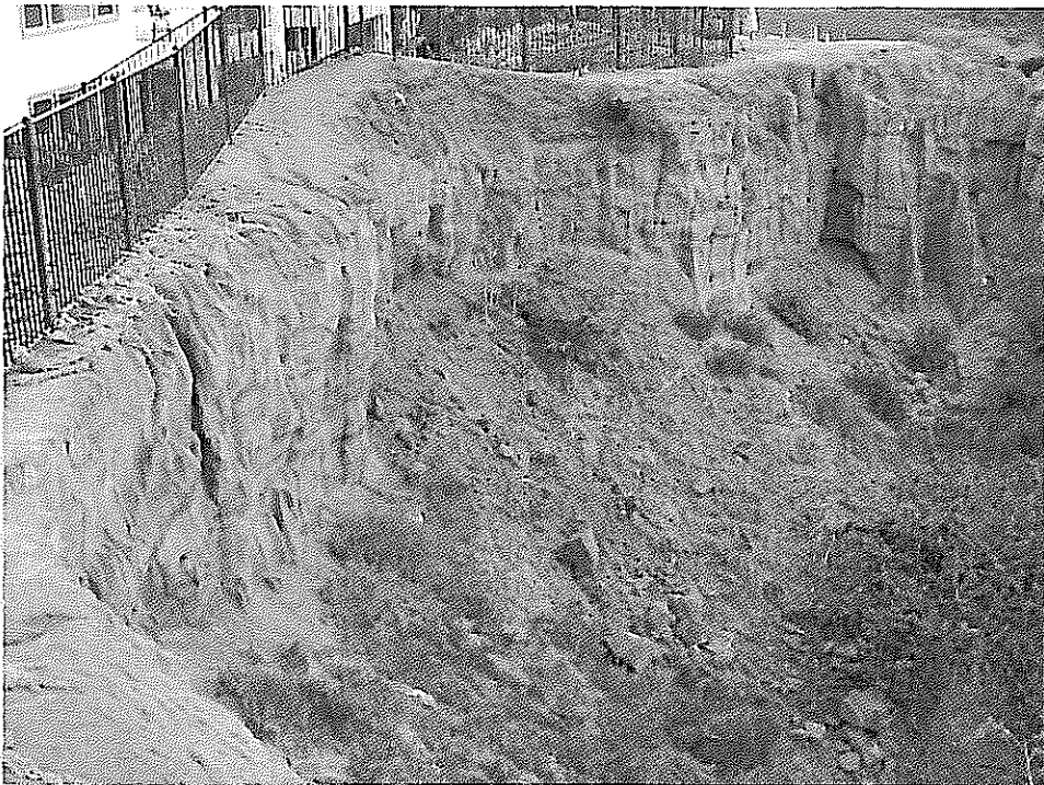
Picture 3. Erosion (fallen soil) along eastern boundary of parcel 208-185-0200. The nonnative plant Myoporum ( Myoporum laetum ) is seen growing through the fence line.
