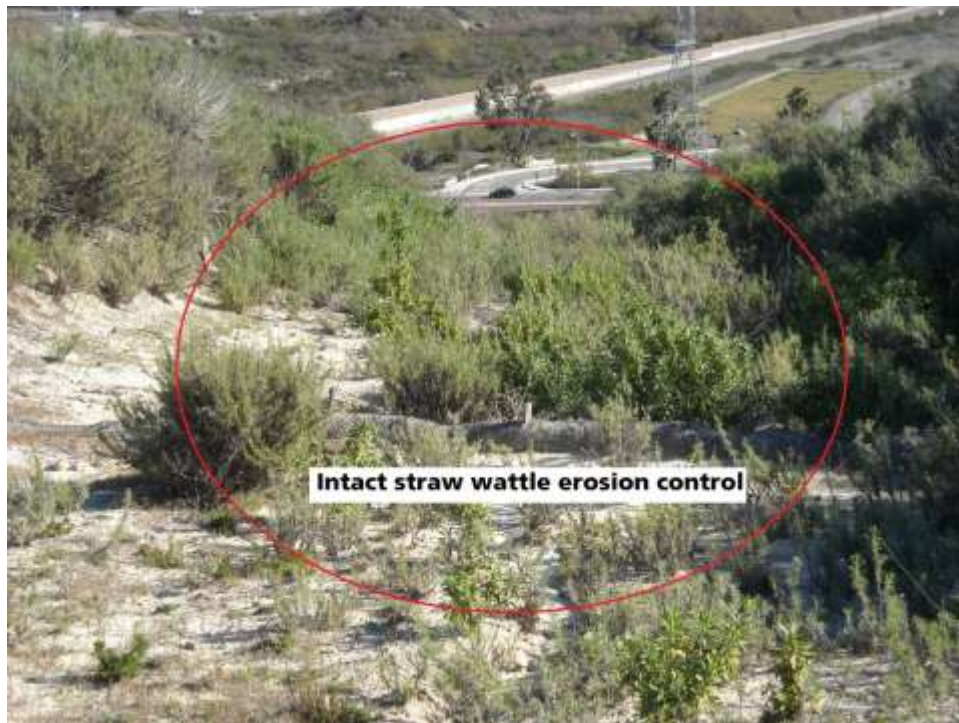
Figure 5 Intact Erosion Control Device
