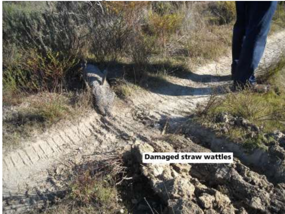
Figure 3 Damaged Erosion Control Device
