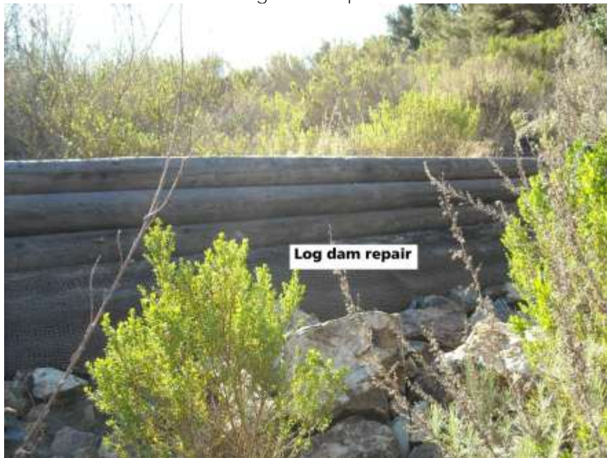
Figure 8 Log Dam Repair
