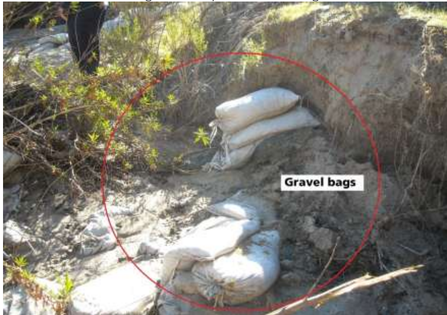
Figure 7 Log Dam Repair-Gravel Bags
