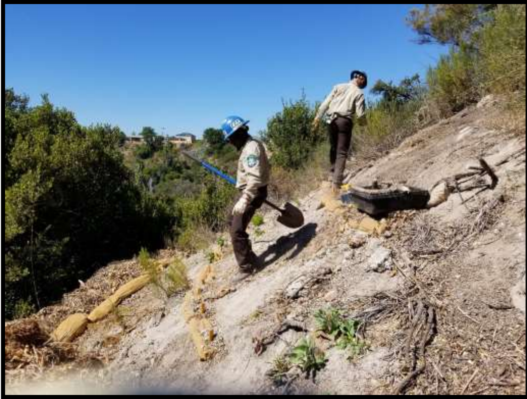
On 10/13/21 CCC crew harvested cactus cuttings and installed them, installed burlap sheets for erosion control and spread seed at Navajo Canyon restoration site. Above picture.
