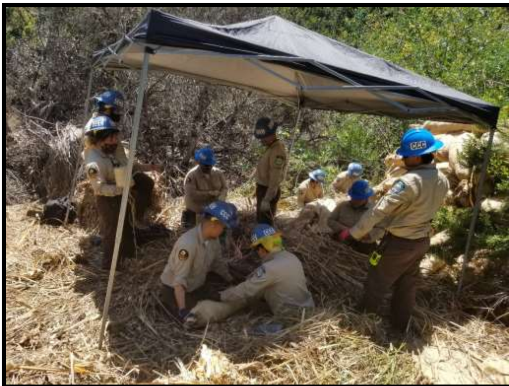
On 5/12/20 - 5/13/20 CCC crew scaled a slope of pampas grass to get to bottom of Navajo Canyon. Crew raked and piled old pampas grass masses into burlap sheets to create pampas grass straw wattles
