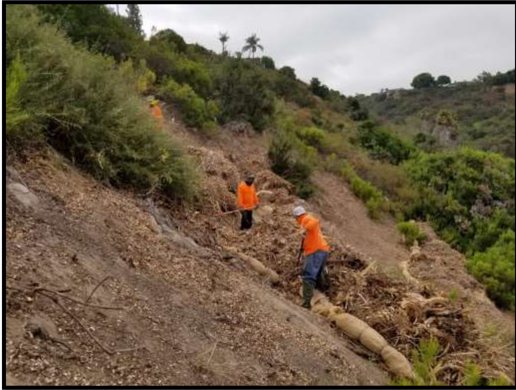
On 7/23/20, 7/27/20 – 7/30/20 Alpha Project crew performed weed control and raked pampas grass biomass into walls and installed hand-made straw wattles (made of burlap, twine and pampas grass biomass) at Navajo Canyon restoration sites. Above picture.
