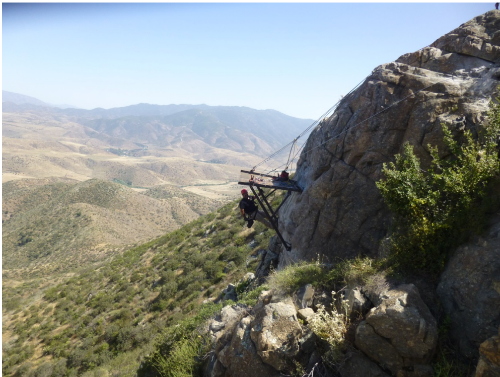
Figure 4. BLM Site installation. Platform in place and bracing being installed. Photo by Frontier Environmental Solutions.
