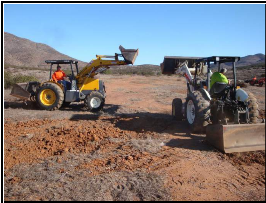
Contractors grading constructed vernal pools.
